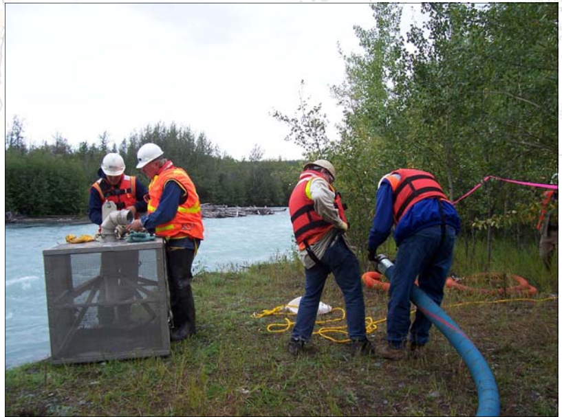
(TOP) Response team preparing fish filter for placement into the Klutina River. Photo taken by Rhonda Williams—JPO/BLM.
